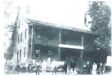
Wheelock Sulfur Springs Hotel dismantled and rebuilt in Peacham
