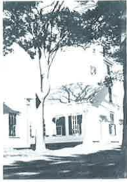
Wheelock Village Church torn down due to disrepair
